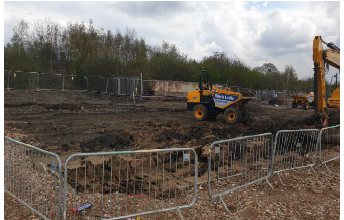
Piling matt installation commenced on 3rd of April for ToC Building
