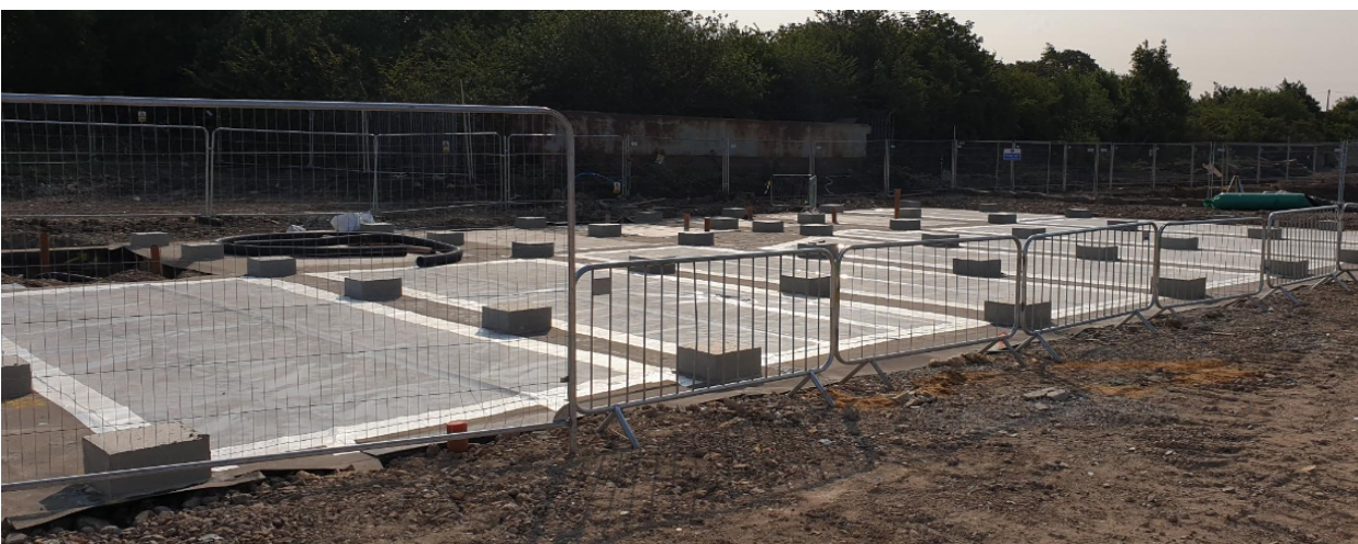
Plinth in readiness for modular ToC building
