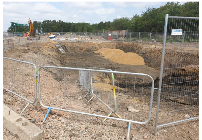
Excavation complete in readiness for attenuation tank 1 installation
