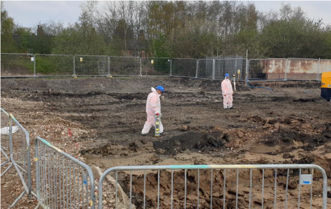
Site Operatives carrying out CAT Scanning to ToC Building footprint
