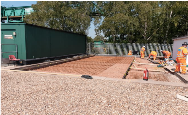
Operatives installing fabric reinforcement to REB (railway equipment base)
