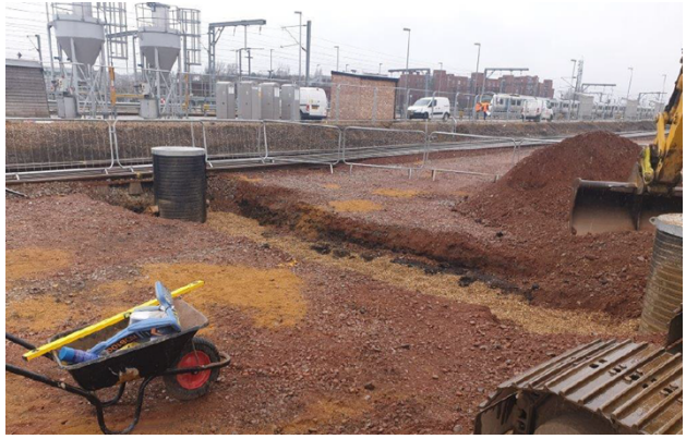
UTX Chambers being installed for lighting Column on Drivers Walkways
