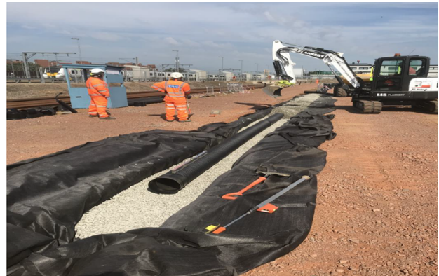
Drainage Run D in South Sidings
