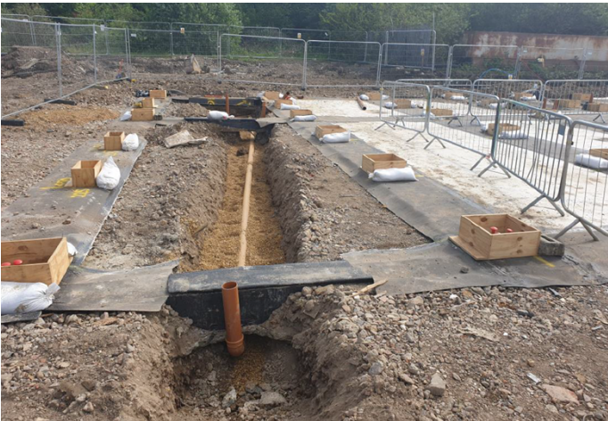
Drainage installation
